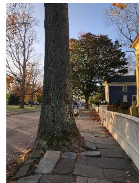
Figure 15 Tuliptree roots in conflict with street, curbing and sidewalk
